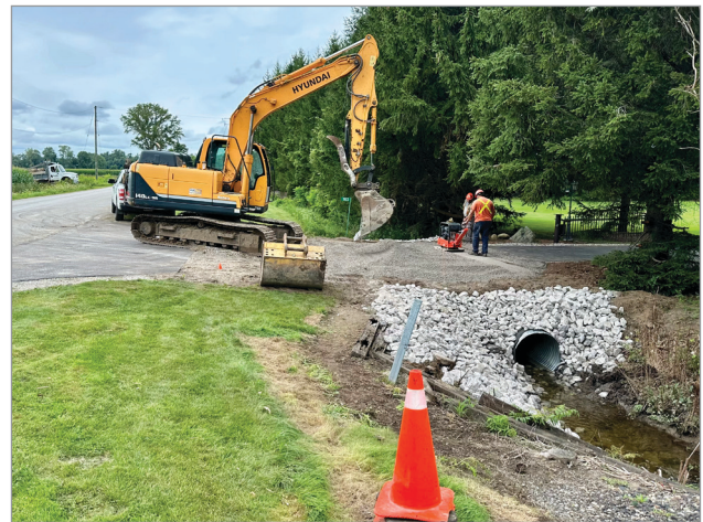
Figure 2. A drain maintenance project.
